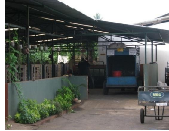
First IRRC Plant
